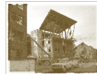
The UW Bothell Library Reading Room under construction.
